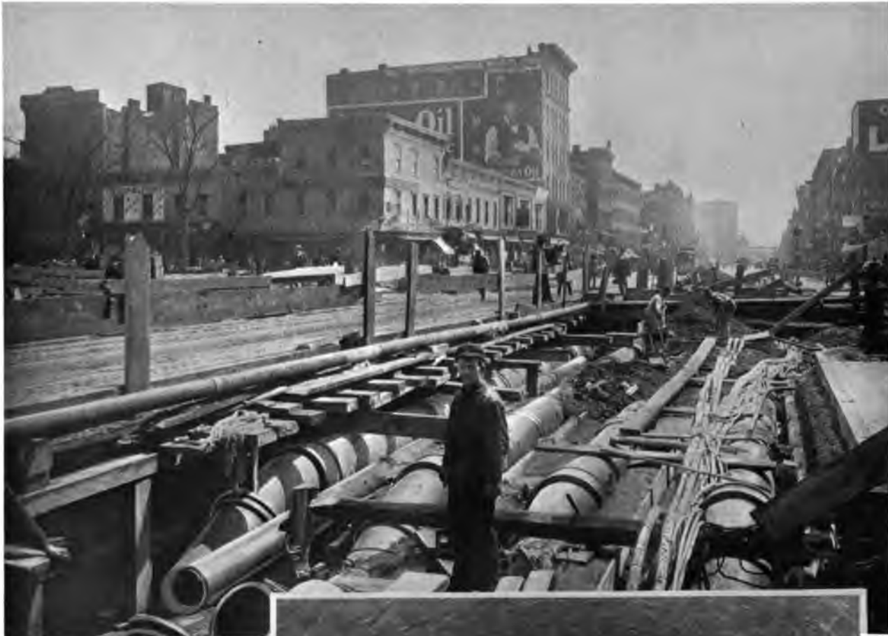
SMALL WATER MAINS BETWEEN STREET SURFACE AND SUBWAY ROOF, SUBSTITUTED FOR ONE LARGE MAIN — 125TH STREET AND LENOX AVE.
